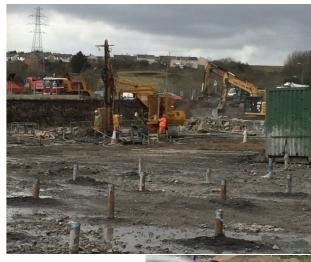
Contract for shallow mine workings consolidation along the route of the A465 Heads of the Valleys road improvements being constructed by Costain in a DBFO contract for the Welsh Government. The project to upgrade 8km of the existing A465 between the Glanbaiden junction at Gilwern and the Brynmawr roundabout to 2 lanes in each direction included a number of areas that were affected by shallow coal workings.
